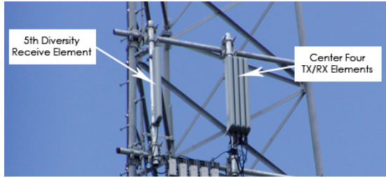
Figure 5 Adaptive Array with Calibration Network
